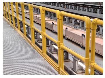
The Fibreglass tube can be quickly cut to length on-site to make the stanchion, handrail and mid-rails with the matched pairs of moulded fittings clamping around the tube to complete all the joints.
