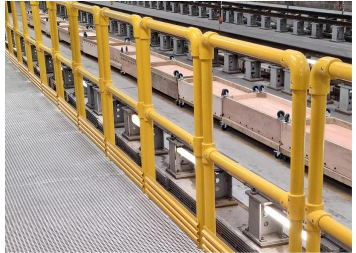
The Fibreglass tube can be quickly cut to length on-site to make the stanchion, handrail and mid-rails with the matched pairs of moulded fittings clamping around the tube to complete all the joints.
