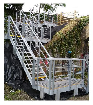
are undertaken by client QTS before being sent to the Step on Safety headquarters in Suffolk. There, the CAD team put together designs that meet all the Network Rail specifications including continuous handrails, anti-slip nosing and self-closing gates.
